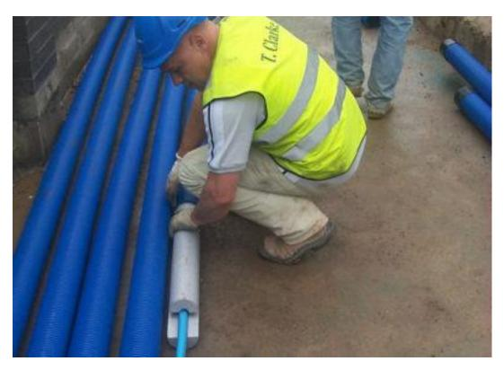
For joints in ducts use proprietary socket joints available through most merchants.
