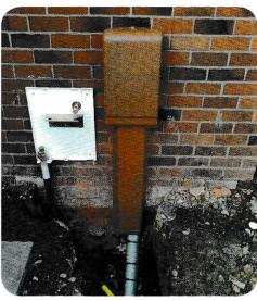
Please Note: the above diagram shows the wall mounted box before the underground ducting was added, ducting will need to be done before you backfill your trench/request an inspection
