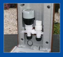
The surface mounted water control management system, allowing metering where traditional installation would be impractical.
