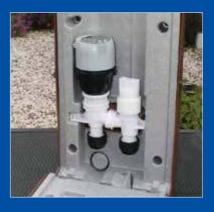
The surface mounted water control management system, allowing metering where traditional installation would be impractical.
